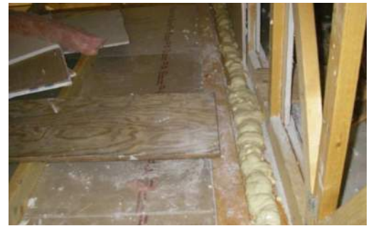
Spray foam installed over top plate joint.
