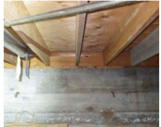
Uninsulated crawlspace interior walls and floor.
