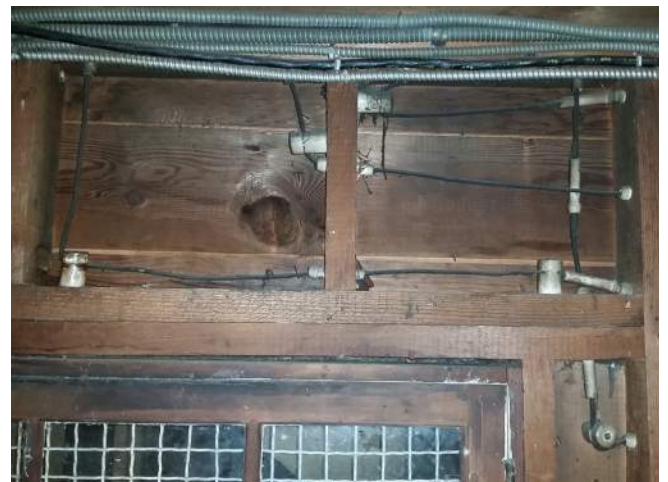
Knob-and-tube wiring.
