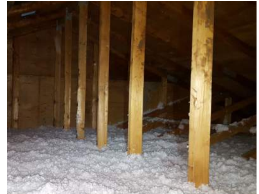
Gable end wall.
