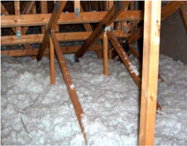
Blown-in attic insulation
