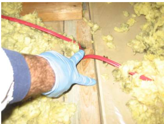
Air sealing of an electrical penetration and unsealed top-plate connection in an attic.
