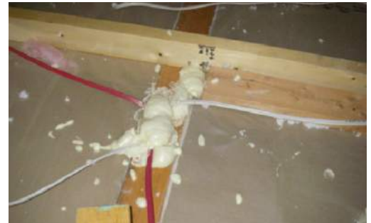
Top plate penetrations sealed with spray foam.
