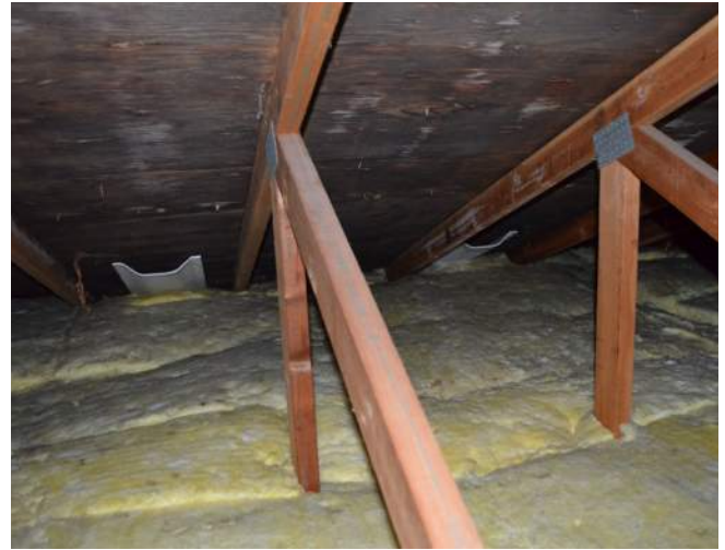
Insulation baffles installed at every second truss bay prior to installation of insulation to provide openings past the insulation from the soffit vents to the attic space.
