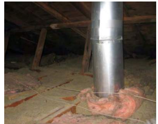
Insulated exhaust duct in attic.
