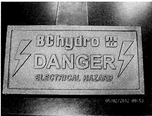
BC Hydro Primary Service Cable Marker Plate
