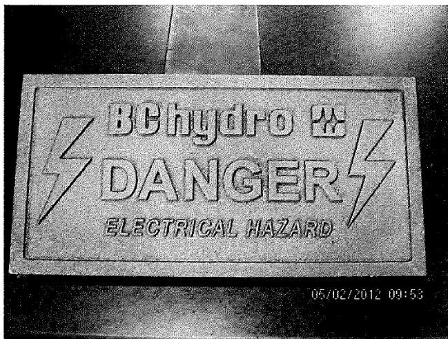
BC Hydro Primary Service Cable Marker Plate
