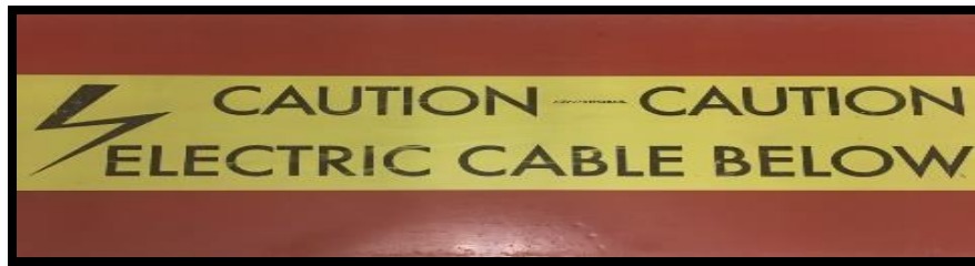
Figure 8-1 – BC Hydro underground duct marker board
