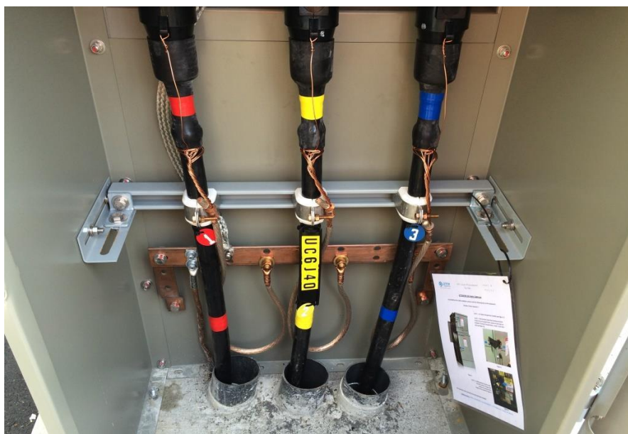
Figure A3-10 – Service cable clamps and adjustable cable support channel
