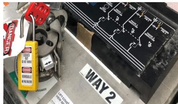
Figure A3-21 – Mnemonic single line diagram and customer locks
