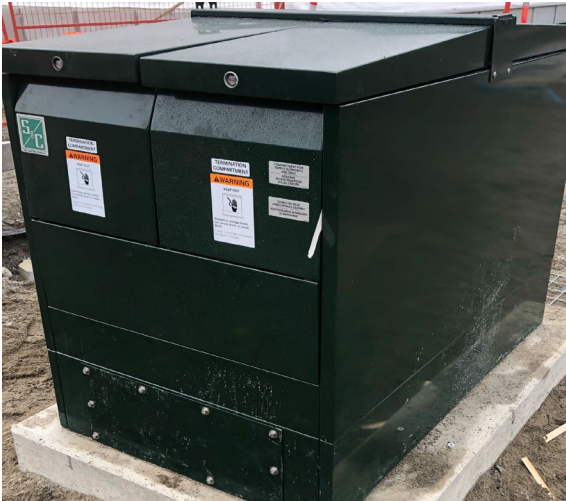
Figure A3-18. Dead-front primary service kiosk by S&C Electric showing BC Hydro as Way 1 and customer service main as Way 2
