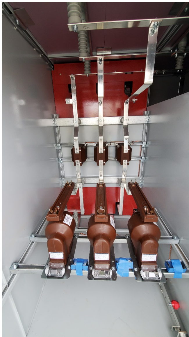
Figure A3-5. Primary revenue metering compartment
