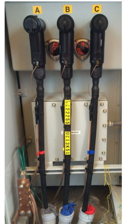
Figure A3-15. BC Hydro utility cable compartment and cable supports and grounding
