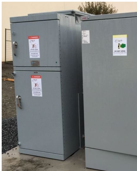
Figure A3-9. Customer-owned dead-front kiosk with both doors closed
