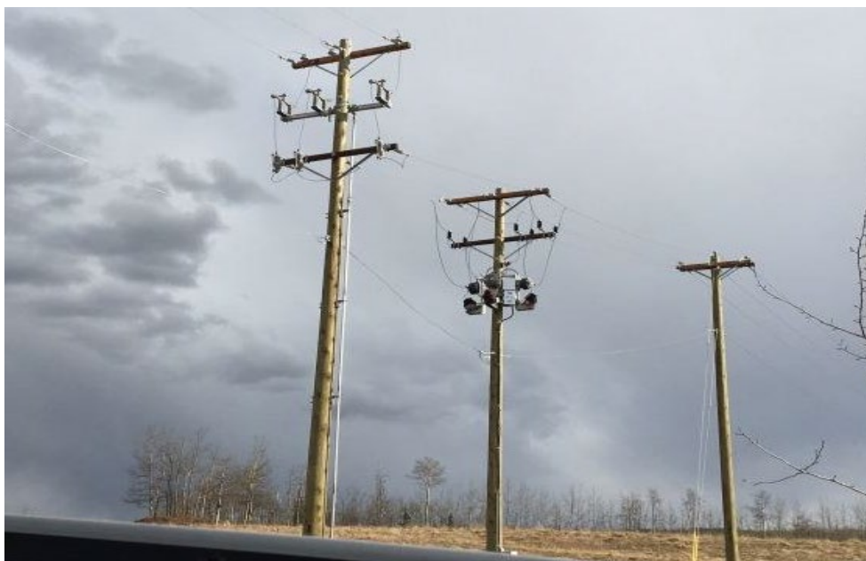
Figure A3-8. Customer service switch and O/C protection on first pole and BC Hydro primary revenue metering on second pole
