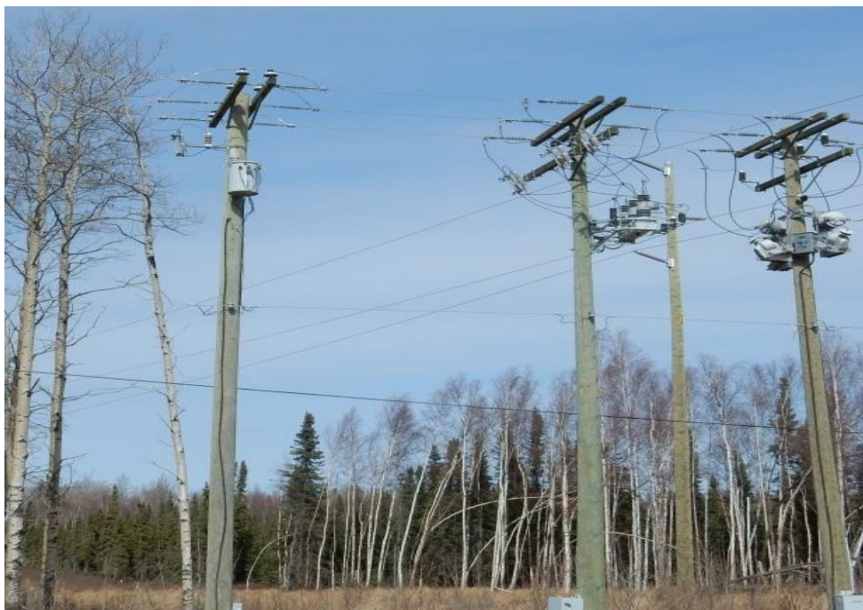
Figure A3-7. Customer-owned recloser and BC Hydro primary revenue metering
