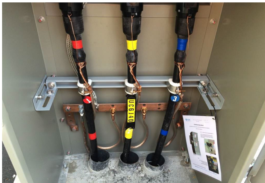
Figure A3-11. Service cable clamps and adjustable cable support channel
