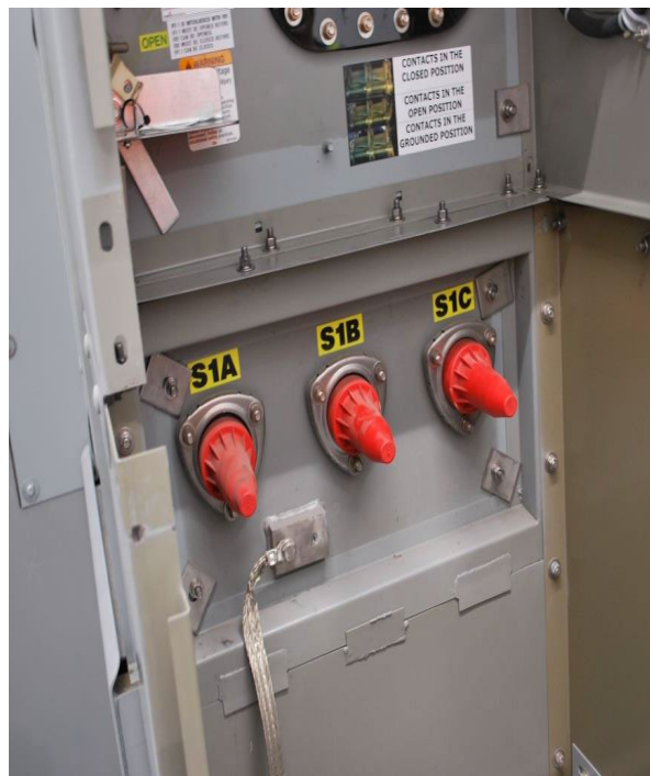
Figure A3-10. Dead-front kiosk both doors open showing grounding switch above and service cable bushings below
