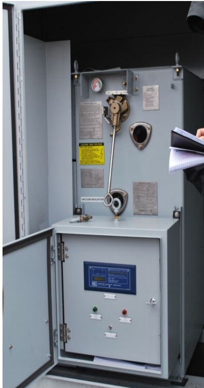
Figure A3-13. Dead front primary service kiosk by Power Systems Technology showing service main
