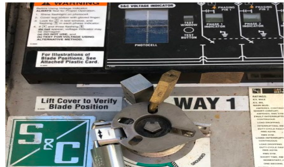
Figure A3-21. BC Hydro grounding position lock
