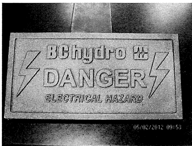
BC Hydro Primary Service Cable Marker Plate
