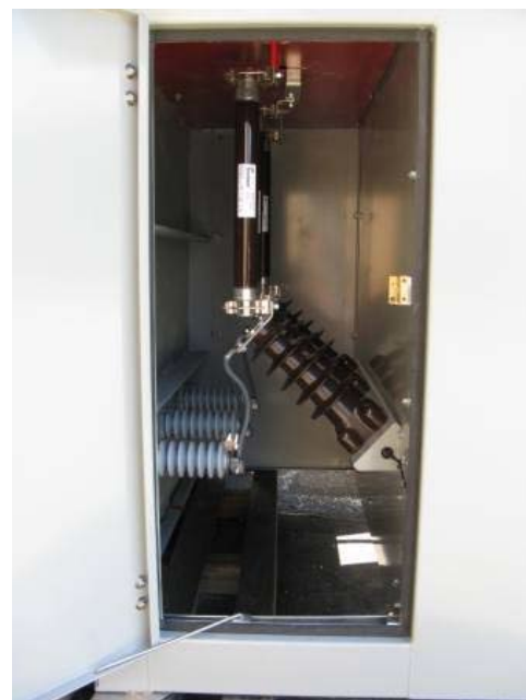
Figure A3-4. Customer-owned primary service fuse compartment
