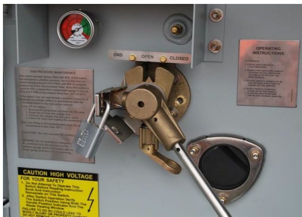
Figure A3-16. BC Hydro grounding position lock
