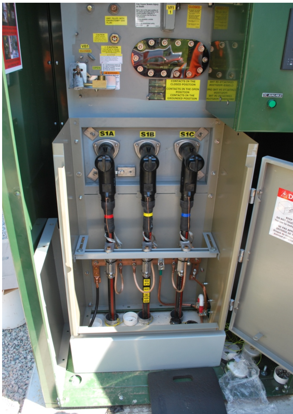
Figure A3-12. Close-up of dead front BC Hydro utility service cable compartment with terminators, cable supports, and grounding
