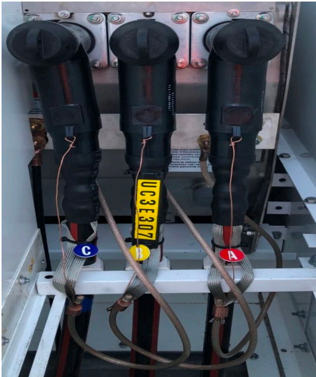
Figure A3-20. BC Hydro utility cable compartment and cable supports and grounding
