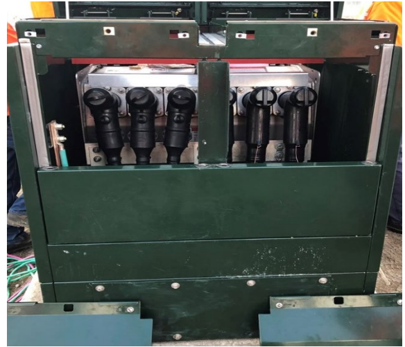
Figure A3-19. Dead-front primary service kiosk by S&C Electric with BC Hydro as Way 1 and customer service main as Way 2, covers open
