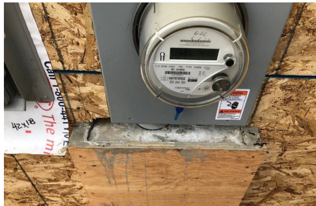
Figure 13 – Concrete encasement bump-out inspection requirement
