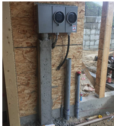
Figure 11 – Concrete encasement not required
