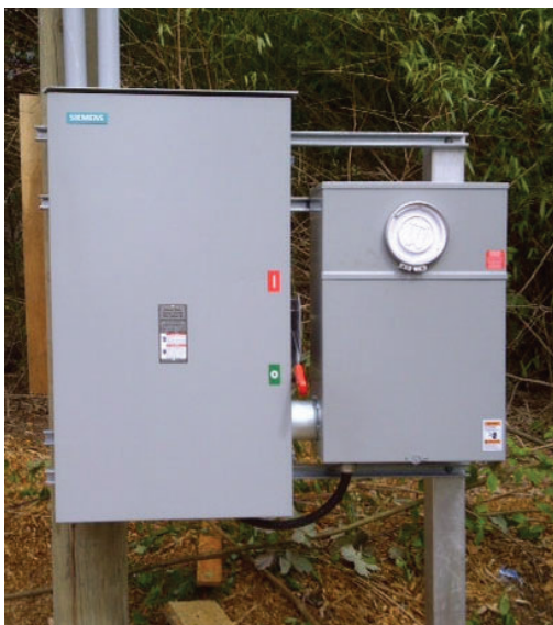
Figure 3 – Unacceptable support structure
