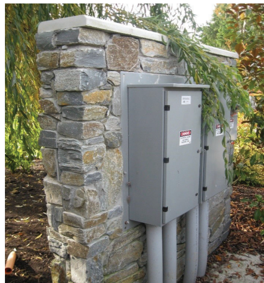
Figure 4 – Acceptable support structure
