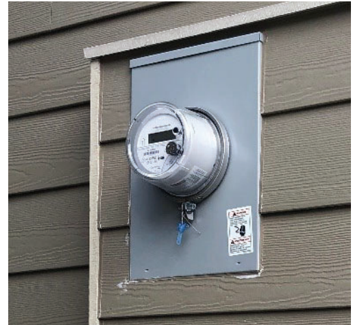
Figure 16 – Unacceptable meter socket without access cavity
