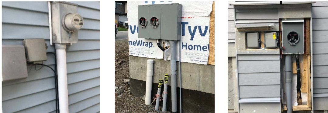
Figure 8 – Acceptable meter sockets installed on wall surface
