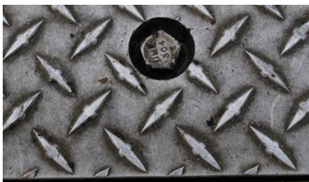
Figure 4 – Aluminum lid with penta bolt
