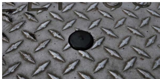
Figure 7 – Puzzle bolt with vinyl cap
