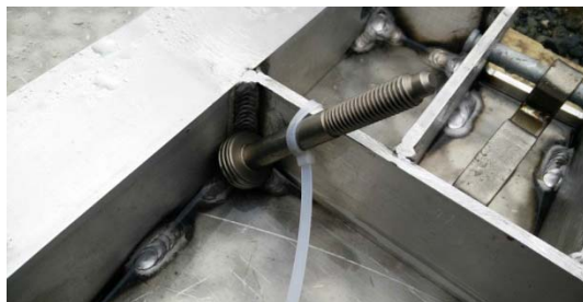
Figure 5 – Puzzle bolt attached to underside
