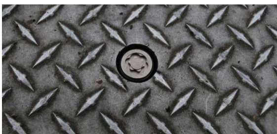
Figure 6 – Aluminum lid with puzzle bolt
