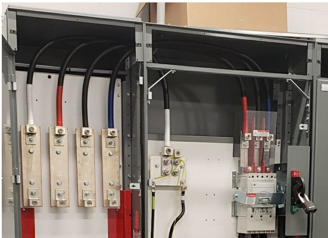
Figure 12 – Acceptable cable bus option for splitter, 100 mm (4") on centre for bus spacing (cable bus from service main breaker terminating into double-sided terminal block inside BC Hydro wireway is unacceptable)
