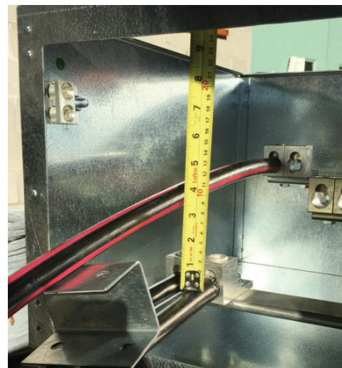
Figure 11 – Phase cables staggered over neutral
