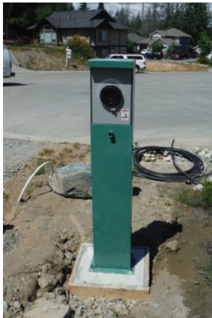
Pedestal with cover installed
