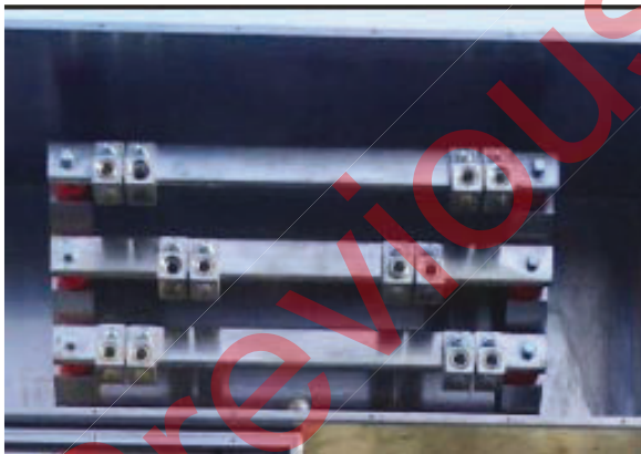
Figure 10 – Splitter bus layout and spacing
