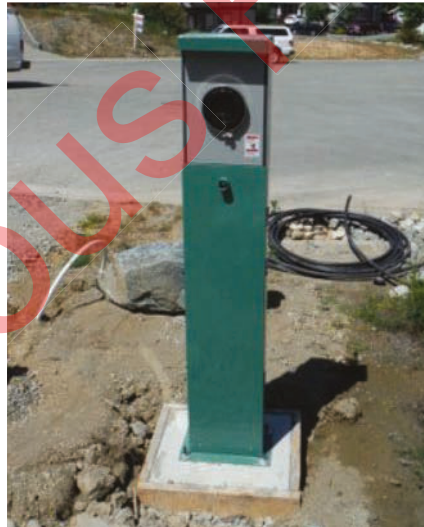
Pedestal with cover installed
