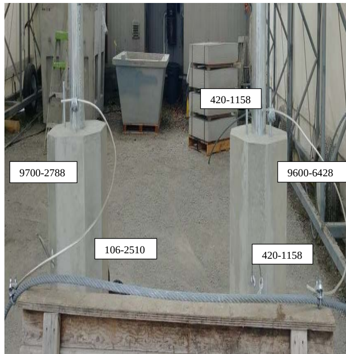
Figure 4 - Precast Bollard Grounding Mock-up
